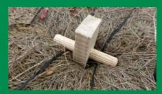
Wooden pins, U-shaped wire pins or steel staples are used for fasten erosion control mats or fabrics. iGGfix offers a large selection a large selection of this mounting gear in various length and designs.
