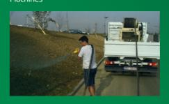
Hydroseeding is a term for a rapid-planting process. A mixture of various seeds and fertilizing components is sprayed over the target area by a machine to be seeded, using a special machine, called the Hydroseeder<sup>®</sup>.
